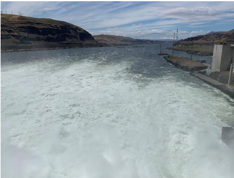
Figure 2. Tailrace conditions. Picture taken from spill gate 3.
